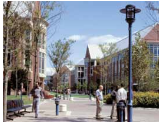
Figure 4 Merrill Lynch Hopewell Campus, Pennington, New Jersey; Architect: Thompson, Venulett, Stainback & Associates (TVS).
