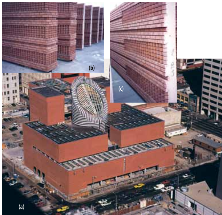
Figure 4 (a), (b) & (c) San Francisco Museum of Modern Art, San Francisco, California; Architect: Mario Botta, Design Architect: Hellmuth, Obata & Kassabaum, P.C. (HOK) Architect of Record.
