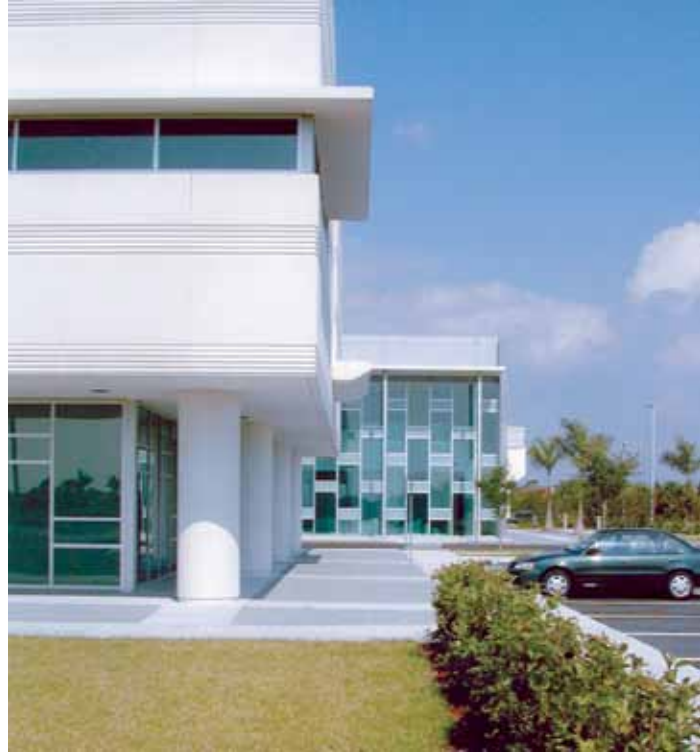
Figure 7 High-reflecting (usually light-colored) surfaces help mitigate urban heat islands. Cape Coral City Hall, Cape Coral, Fla.; Architect: Spillis Candela/DMJM.
